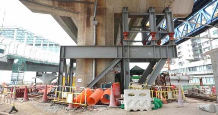
Temporary support for the re-aligned pier head for the servicing Island Eastern Corridor
