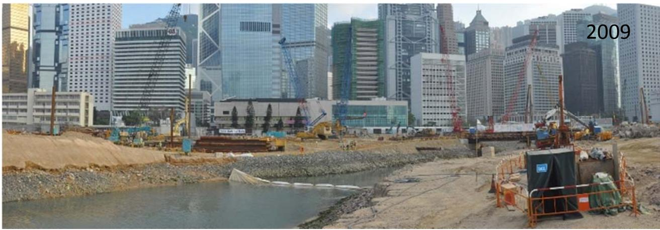
One of the most difficult work for reclamation work – diversion and extension of the storm water discharge culvert.
