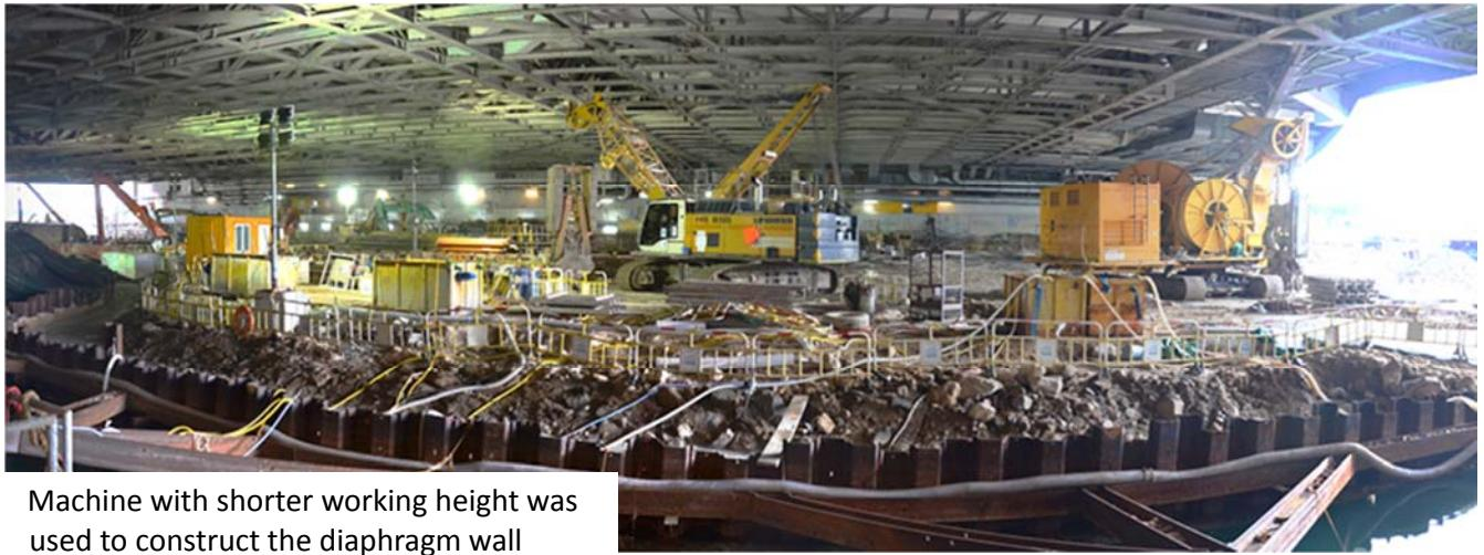
Machine with shorter working height was used to construct the diaphragm wall
