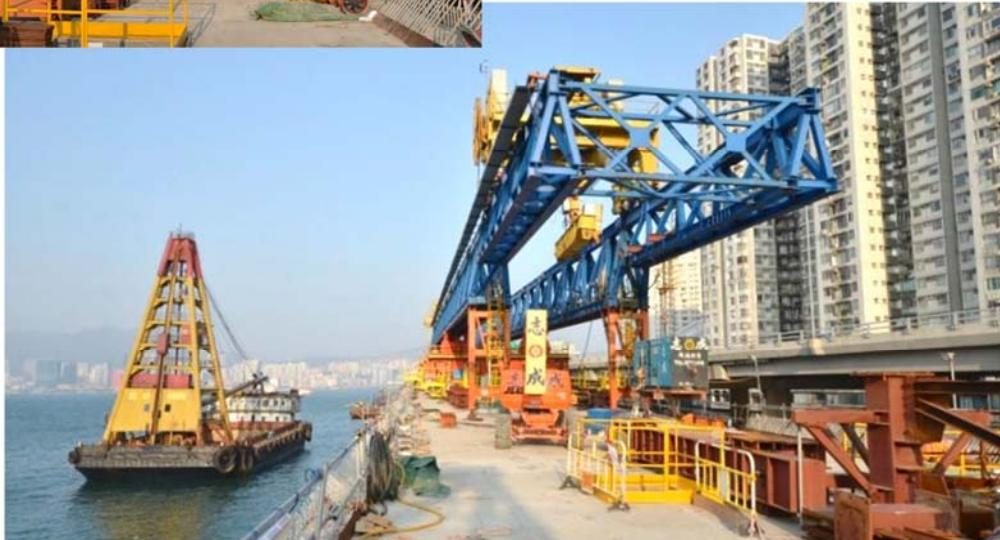
The two sets of launching gantry used in the North Point Interchange section
