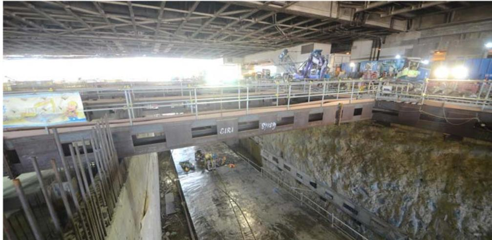
Semi-top method to construct the carriageway tube
