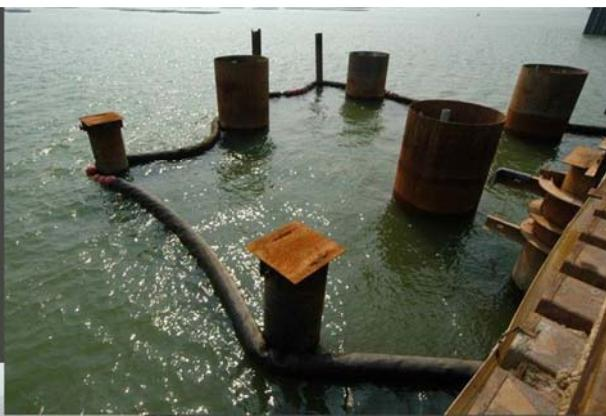
Provision of silt screen to confine silt and marine mud
