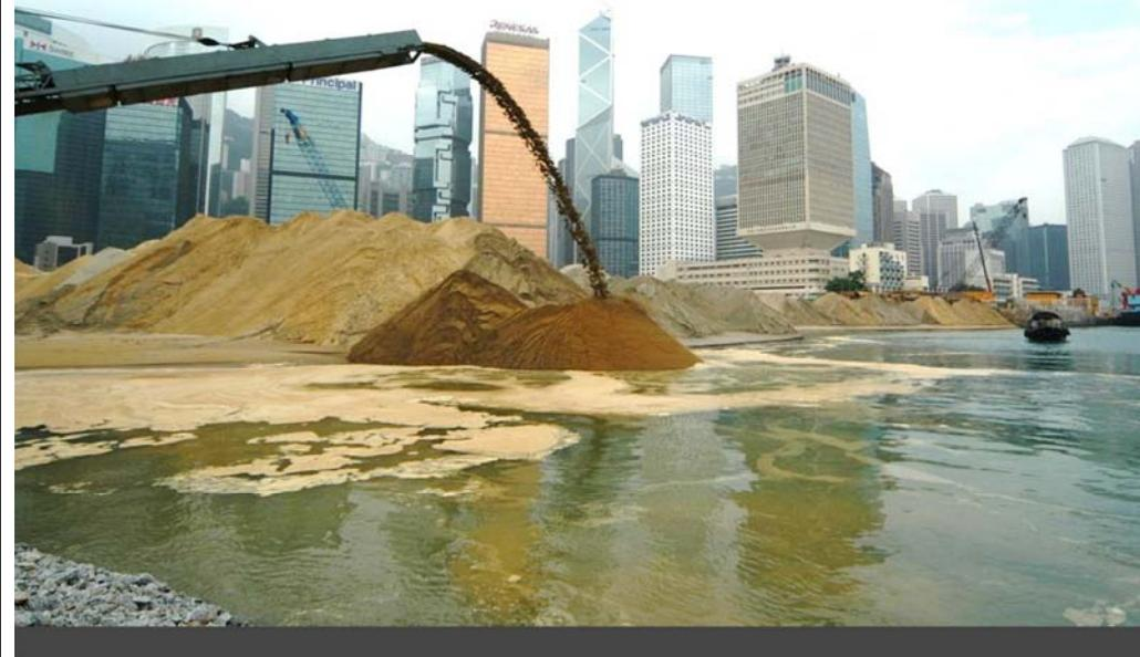
Reclamation by sand-filling using conveyor belt or pump
