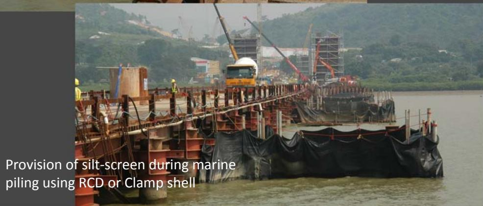
Provision of silt-screen during marine piling using RCD or Clamp shell
