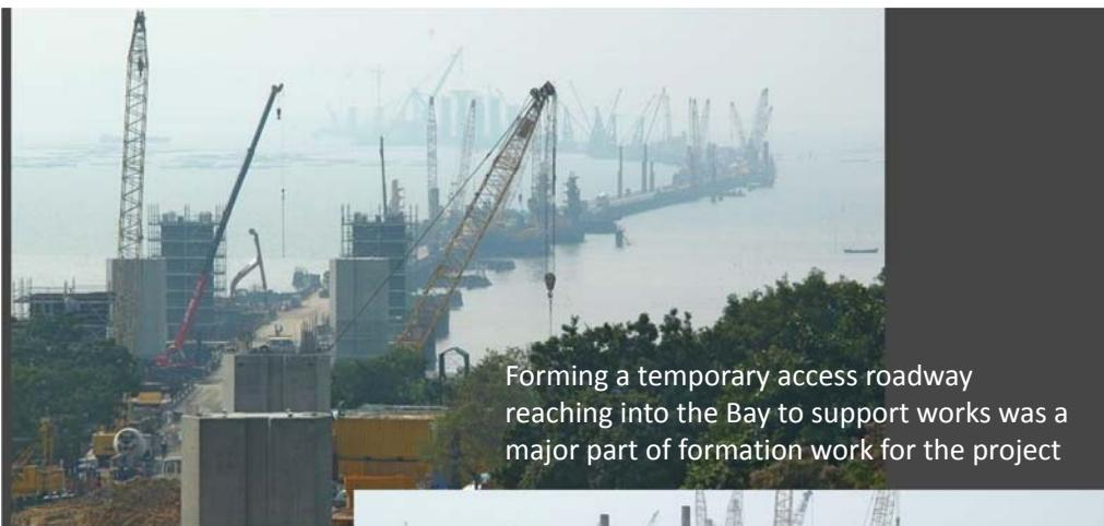
Forming a temporary access roadway reaching into the Bay to support works was a major part of formation work for the project
