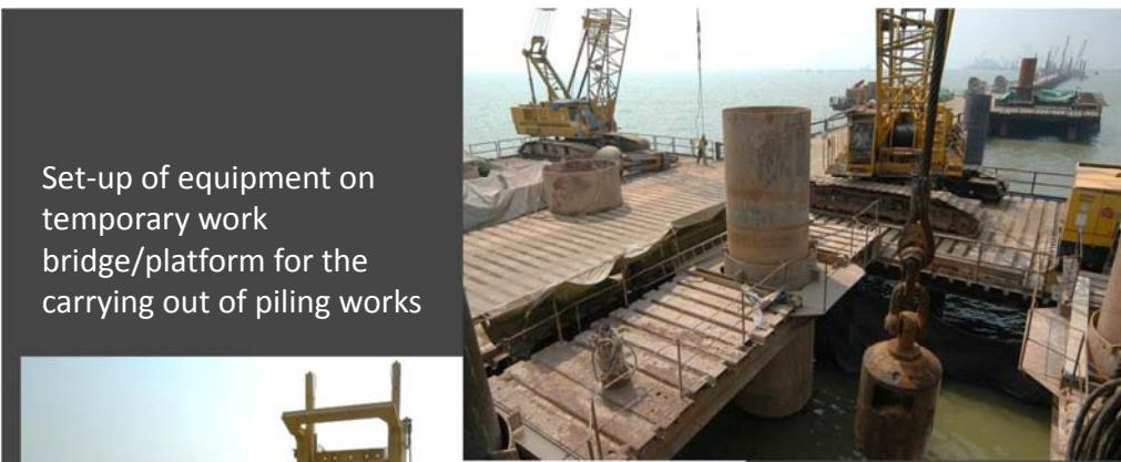
Set-up of equipment on temporary work bridge/platform for the carrying out of piling works
