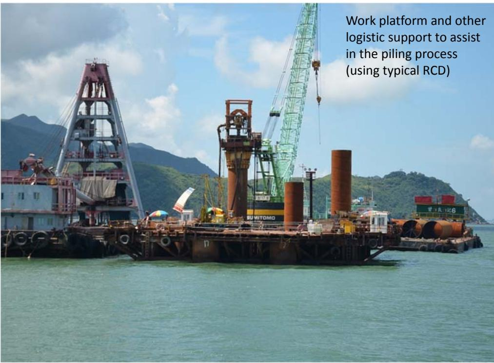
Work platform and other logistic support to assist in the piling process (using typical RCD)
