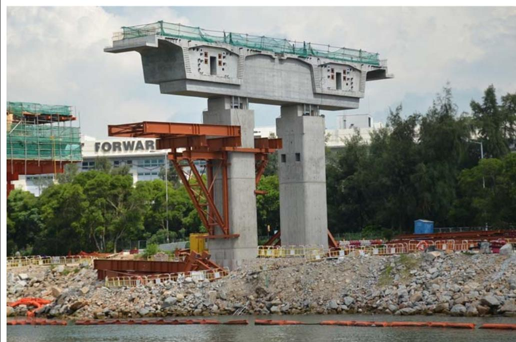
A typical portal beam for dual-way 3-lane carriageway
