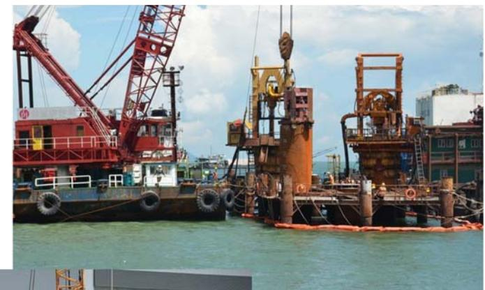
Setting-up of the RCD for the formation of the bore-piles
