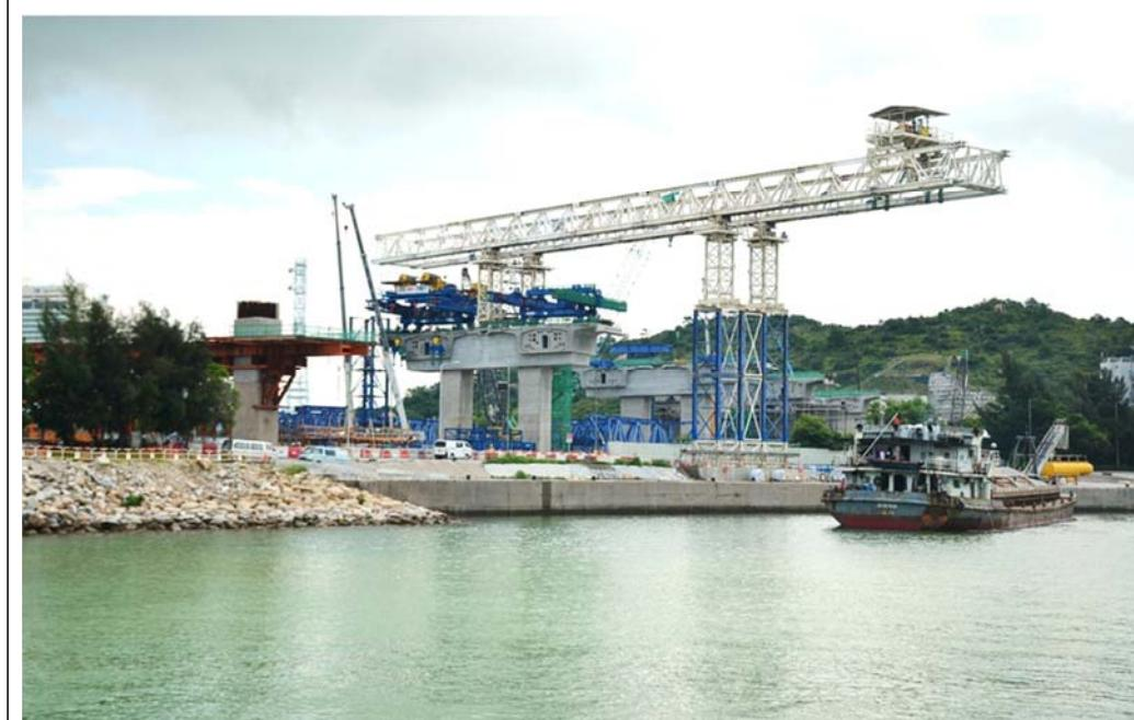
Loading and preparation yard to support the construction of the viaduct (handling precast segments)
