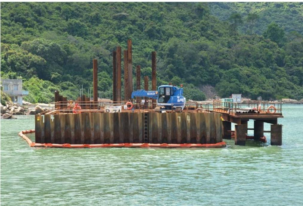
Using of sheet-pile to form a water-sealed cofferdam for the forming of the raft cap
