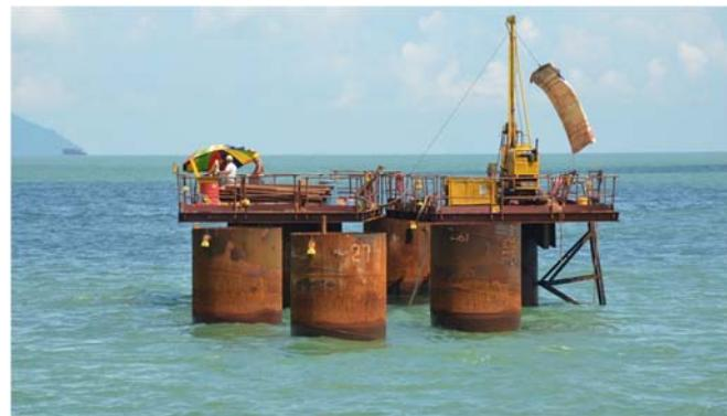
Typical setting of work platform for the on-going works (forming the raft-cap and piers)
