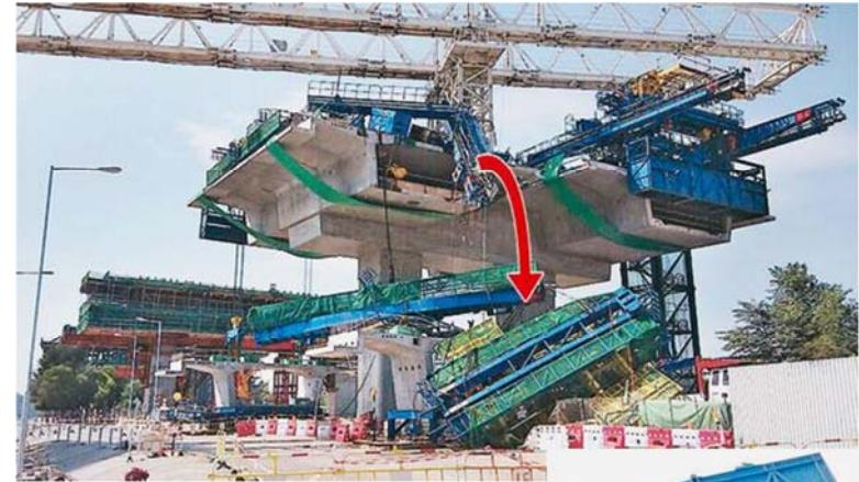
An accident happened in 2014 – collapse of the launching gantry for the erection of the precast girder for the viaduct.
