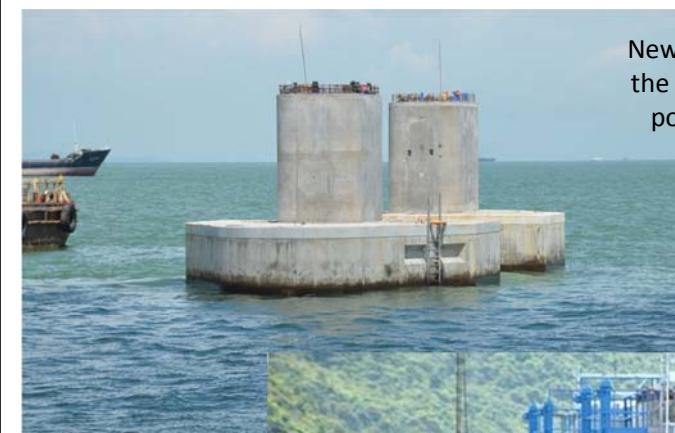
Newly completed raft cap with the first section of pier for the portal beam being in place
