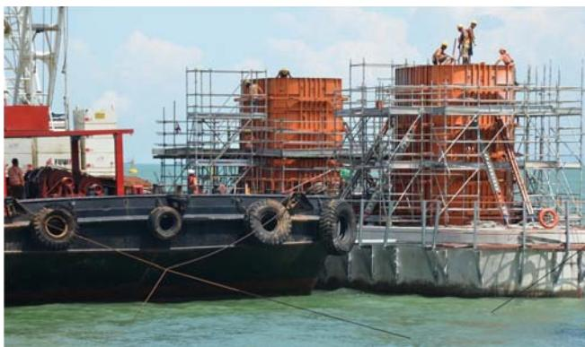
Forming the pier using typical steel gang-form
