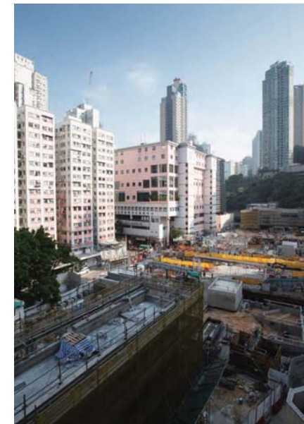
Kennedy Town Station Site on West Island Line
