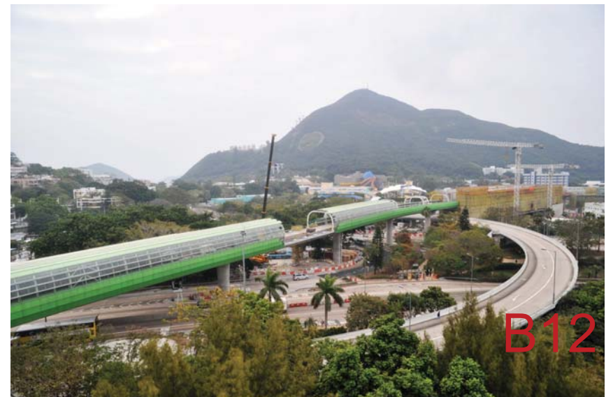
South Island Line (East) Viaduct Section
