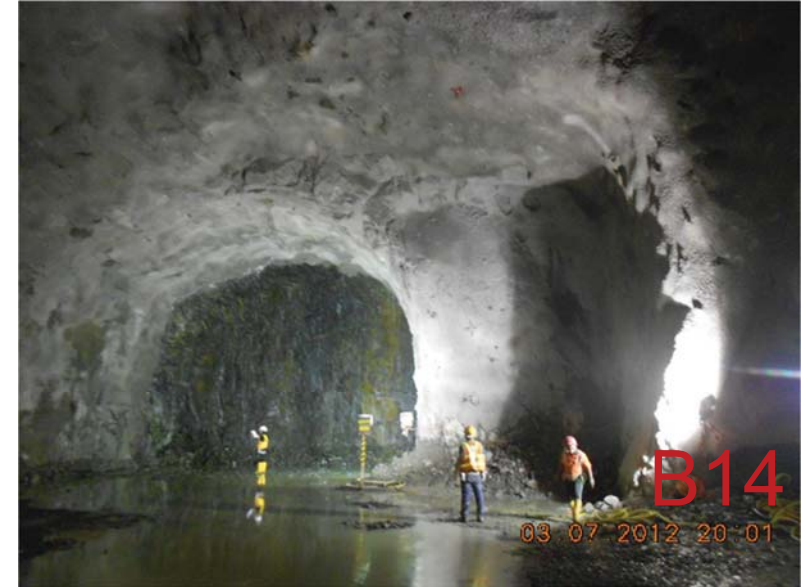
Drill and blast tunnelling for SIL(E)
