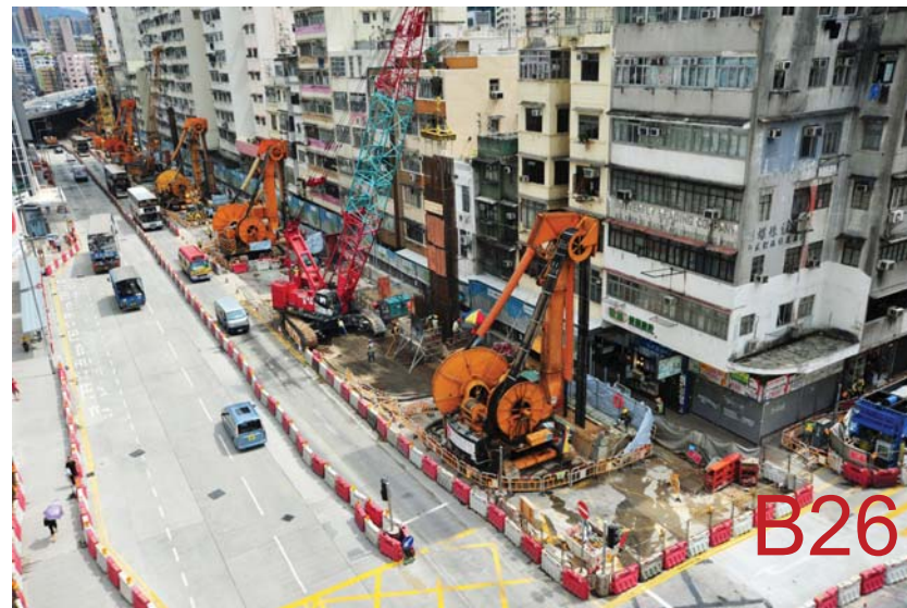
Diaphragm wall works for Ma Tau Wai Station of SCL EWL
