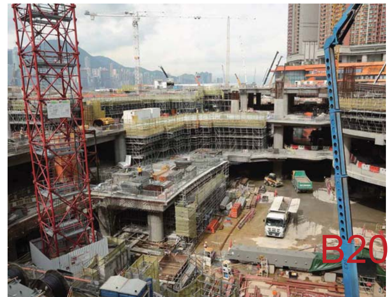
West Kowloon Terminus concrete works
