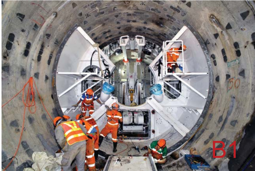
Innovative Tunnel Dismantling Machine used on West Island Line
