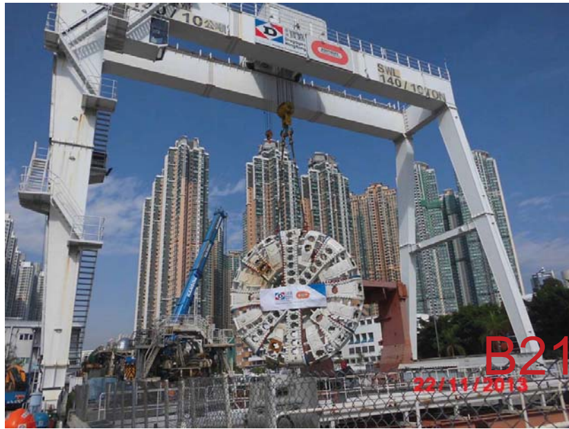
Lifting a TBM Cutter Head for XRL southern section tunnel
