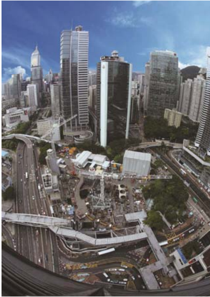
Harcourt Garden Site-Admiralty Station works for SIL(E) and SCL NSL
