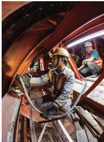
Railway tunnel lining construction for West Island Line
