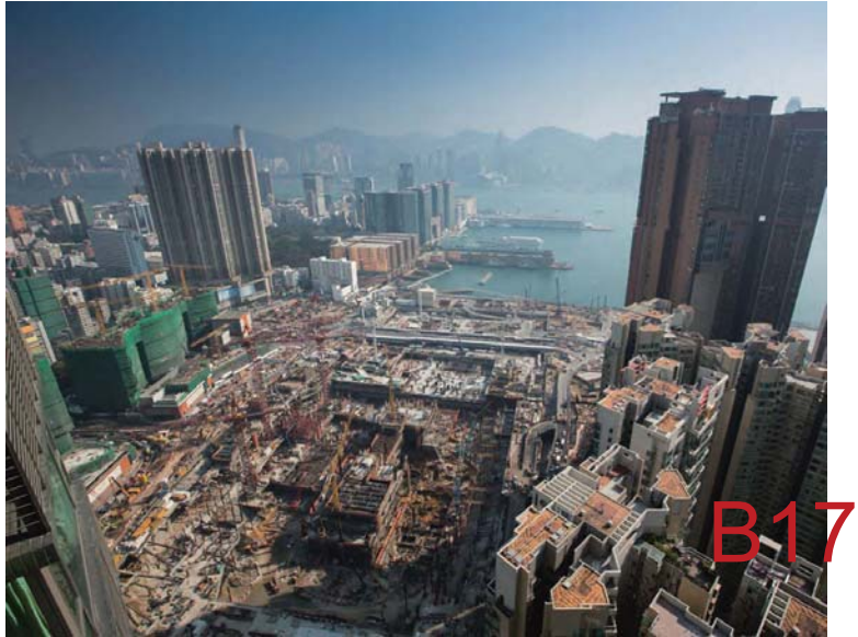
West Kowloon Terminus site for future Express Rail Link
