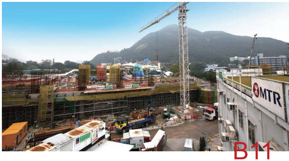
Ocean Park station construction for South Island Line (East)
