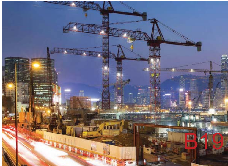
Cranes and skyscrapers-Twilight at West Kowloon Terminus
