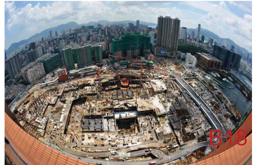
West Kowloon Terminus construction
