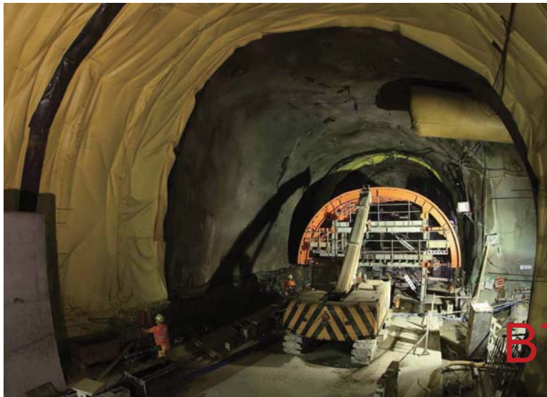
Tunnel lining works at future integrated Admiralty Station
