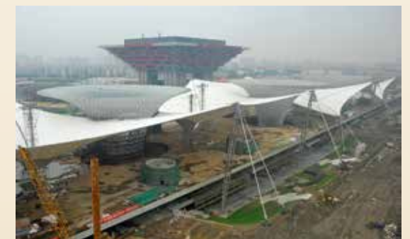
▲ Construction of the China pavilion for the 2010 Shanghai World Expo.
