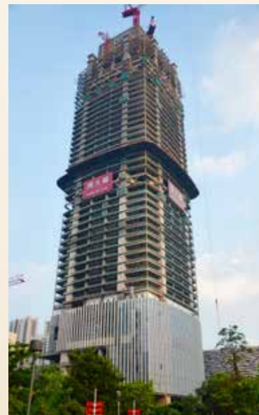
▲ Construction of the Chow Tai Fook Tower as seen in 2012.
