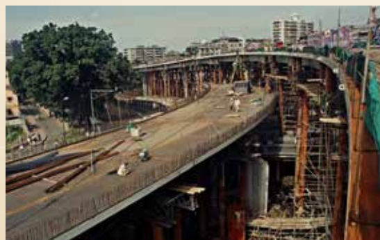
▲ Construction of the Inner Ring Road near Shamian, Liwan (1998) (沙面·荔灣區)
