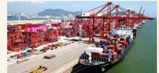
▲ An overview of Yanshan Deep-water Port.
