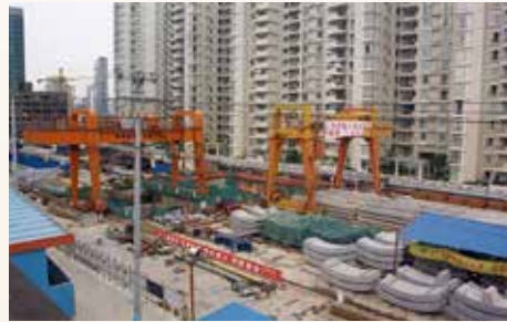
▲ Construction of the Metro Line 9 at Xujiahui (徐家匯)
