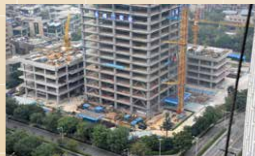
▲ Construction site is maintained relatively quite in order and tidy nowadays.
