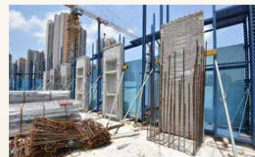
▲ Use of precast elements in building construction is becoming popular
