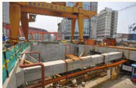
▲ Construction of the Metro Line 12 at Hong Kou (虹口)
