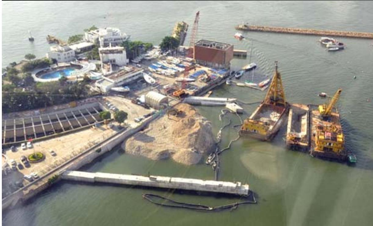
Temporary reclamation and construction of SCL tunnel in Causeway Typhoon Shelter
