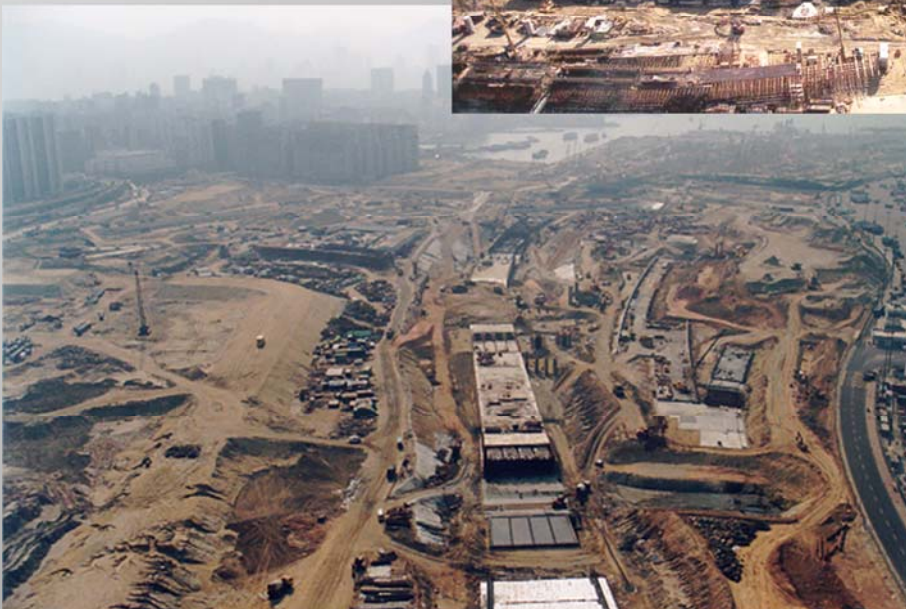
Construction of the Kowloon Station and the cut-and-cover tunnel of the Airport Railway at its early stage in 1995
