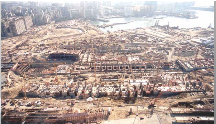
Construction of the Kowloon Station and the cut-and-cover tunnel of the Airport Railway at its early stage in 1995
