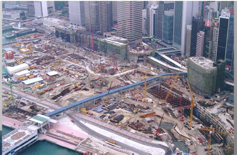
Cut-and-Cover Tunnel for the Airport Railway in the newly Reclaimed Land in Central
