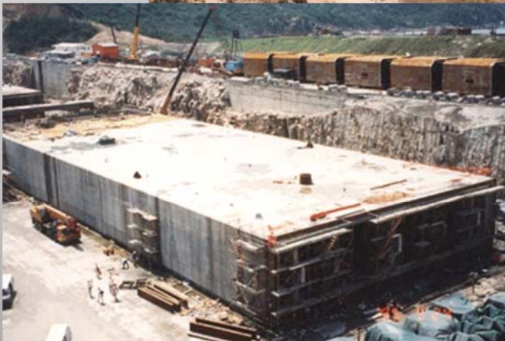
Casting yard for the forming of the submerge tunnel tubes at Shek O Quarry
