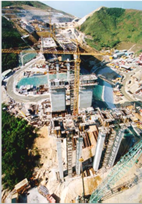
Forming the approach section of the KSM Bridge on the Lantau side
