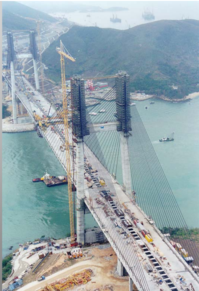
Kap Shui Mun Bridge – a 430m cable-stayed bridge
