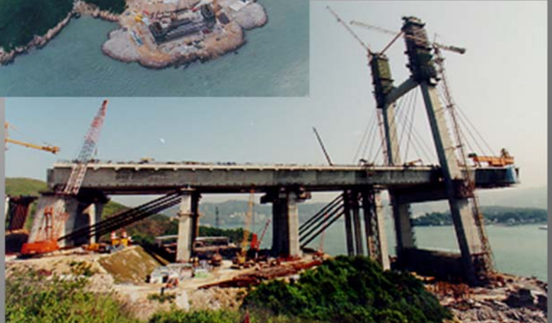
Forming the approach section of the KSM Bridge on the Lantau side
