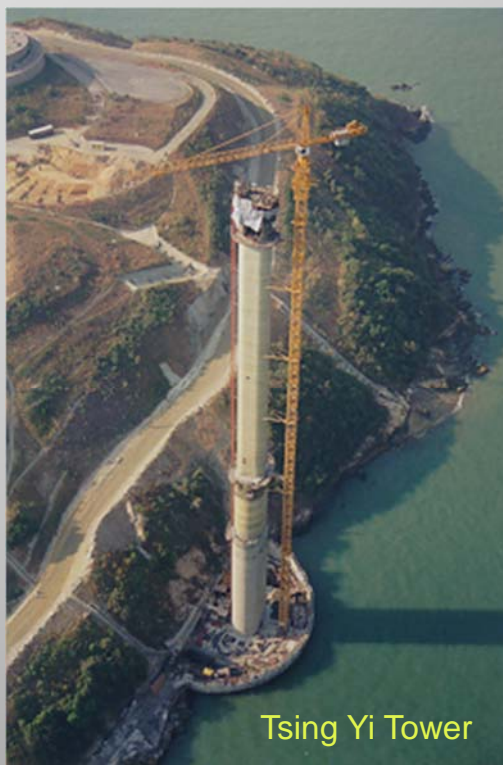
Construction of the bridge towers
