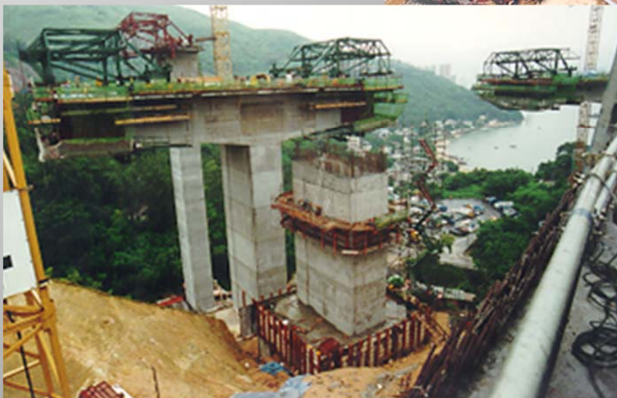
Construction of the approach viaduct using balanced cantilever method (traveling form)
