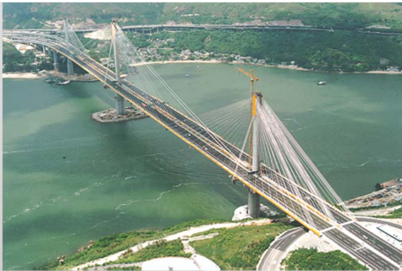
Ting Kau Bridge is a cable-stay bridge in 3 spans
