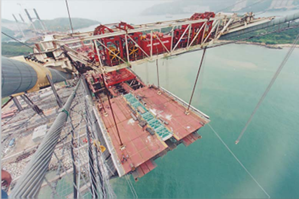
Close up of the lifting gantry that mounted onto the main cable for the lifting and temporary positioning of the prefabricated deck
