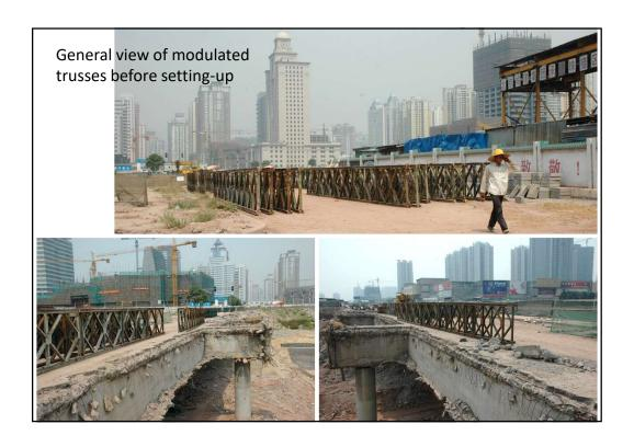
Using modulated trusses to form a temporary pedestrian footbridge
