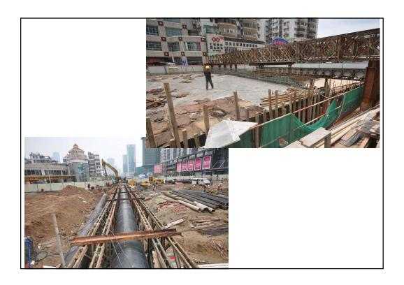
Examples of using modulated trusses to set up the falsework system to construct a bridge by incremental launching method (Leide Bridge in Tienho, Guangzhou 廣州天河腊德橋)
