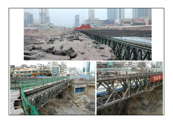
Closer view of some of this temporary utility support in the form of a continuous simple truss bridge
