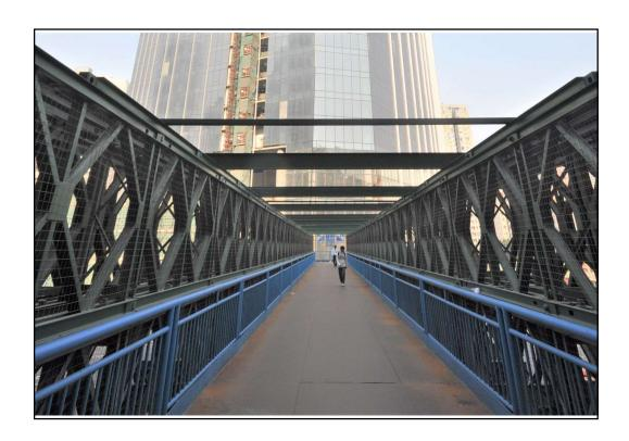
Use as temporary roadway linking up disturbed servicing roadways to allow large area of excavation
